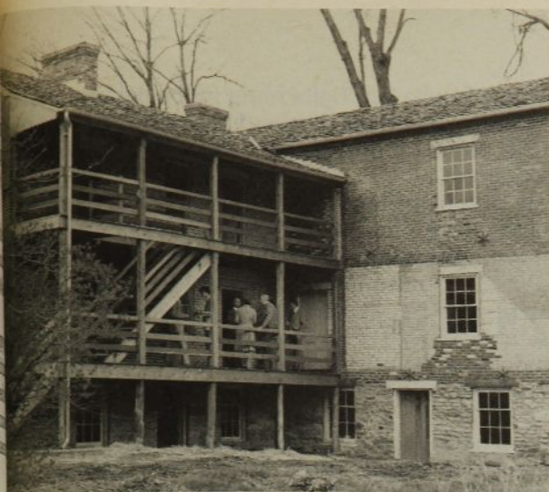
Evidence indicates that the Founders House was constructed in the early 1850's upon the foundation of an old tavern or inn. The foundation is from local limestone laid up in lime mortar and is amazingly thick, being 24 inches thick at the base and tapering to 18 inches. Inner linings of brick rise directly from the limestone foundation. Brick was chosen for the Fraternity's birthplace because of its great availability in Bethany.
